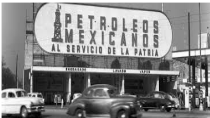
Figure 1: Old filling Pemex station, 1956, from Fortune Magazine
